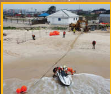
Landing stations: bringing subsea cables ashore.
